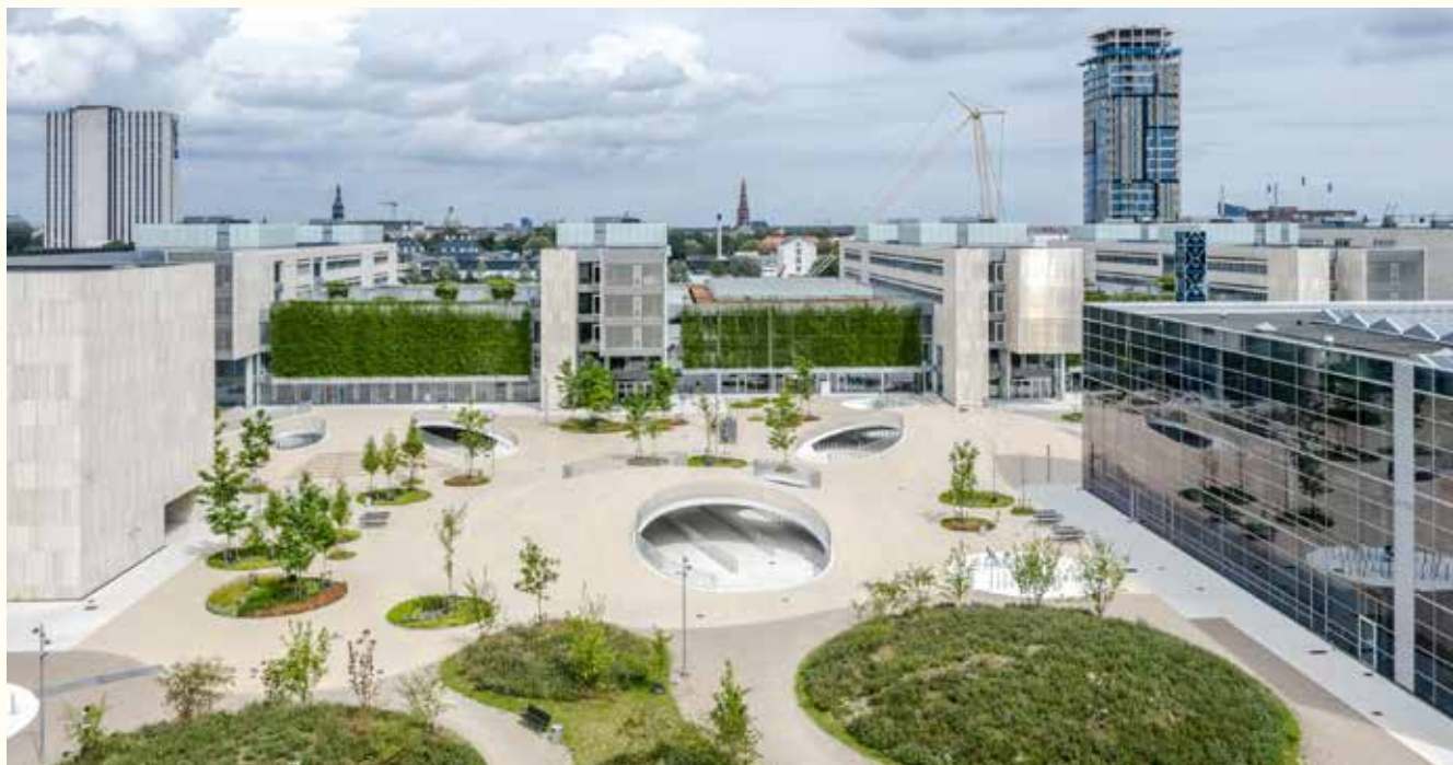
Karen Blixens Square at the University of Copenhagen. Bicycle shelters and plant beds are built to retain water. Image credit: Cobe
