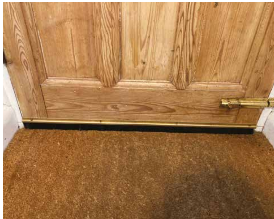
Draught proofing strip fixed to bottom of external door
