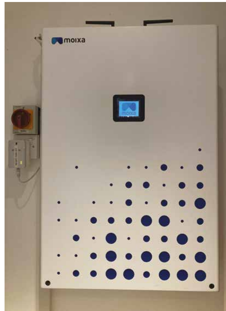
Wall mounted solar battery
