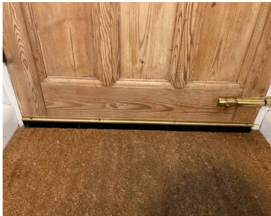
Draught proofing strip fixed to bottom of external door
