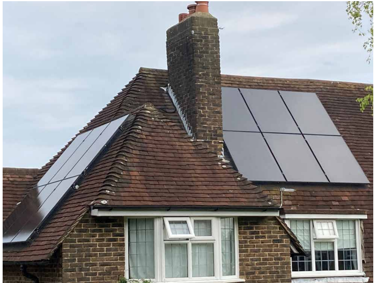
Solar panels on south and west facing roof slopes
